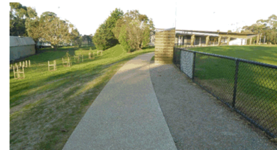
New exposed aggregate path to perimeter of Oval 1
