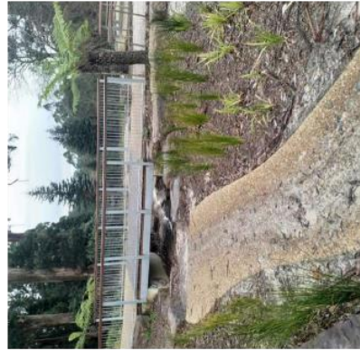
Concrete-lined swale with bridge crossing
