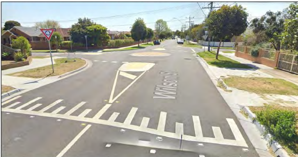
Figure 8 Example of a raised treatment at a roundabout (from Google Maps Streetview)
