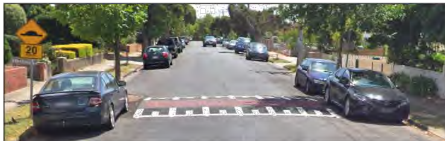
Figure 5 Example of a speed hump (from Nearmap aerial photography)
