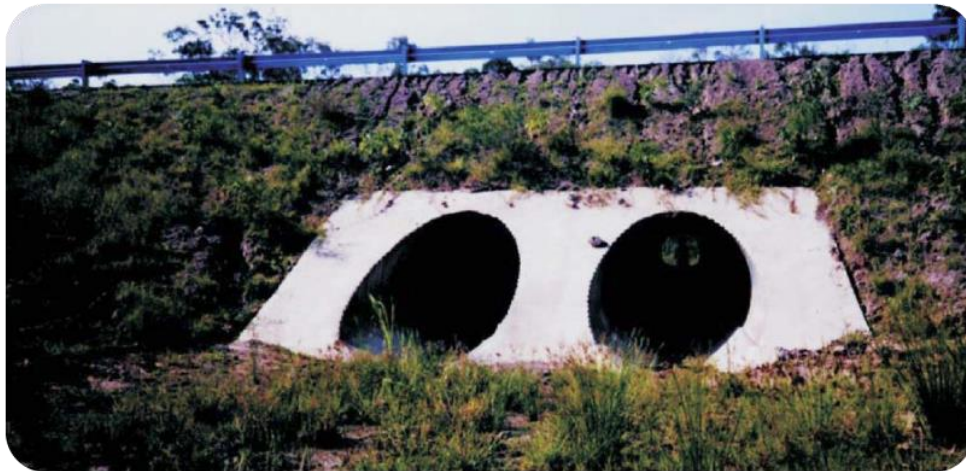
Image 20. A large culvert under a freeway, which is a great passage for ground-dwelling fauna. Photograph from Queensland Department of Main Roads (2000).
