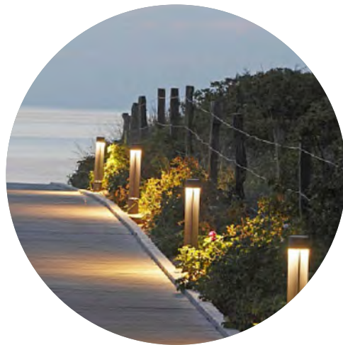
Underground power for pedestrian focused lighting
