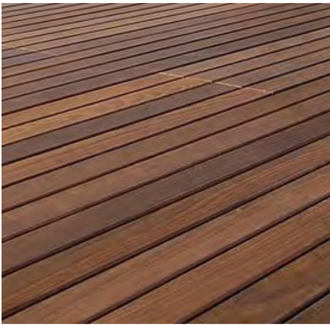
Specialised Zones Timber surfaces
