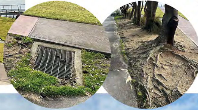
Realign paths away from compacted tree roots (trip hazard, but also long-term risk to tree survival).
