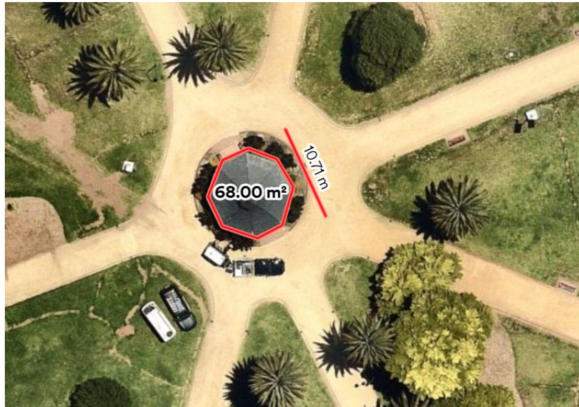
Image (Above) – Bicentennial Rotunda, Catani Gardens, St Kilda – Structure footprint
