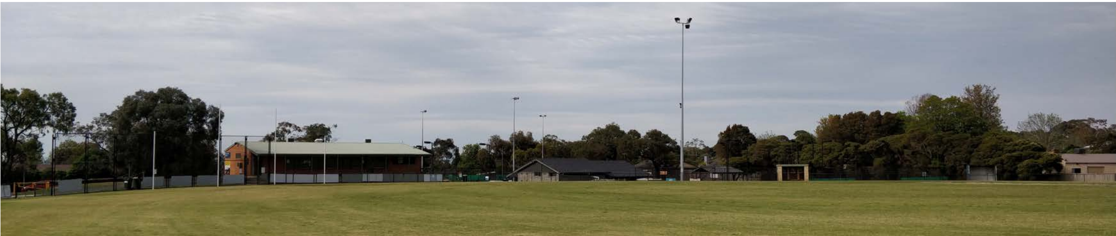
Above - View from parking overflow (looking north)
