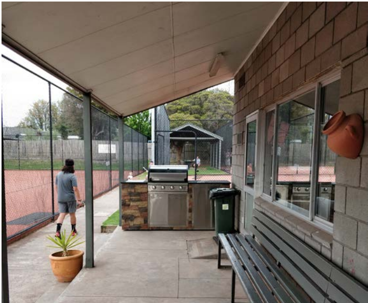
Above - View of tennis pavilion covered way (looking east)
