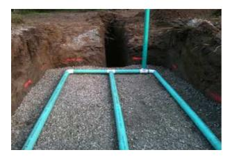
The concrete pit at the start of the sand filter is generally square in shape, and is referred to as the distribution pit or box. If you lift the lid of this pit and look inside, you will see a round opening on each of the four walls of the pit. All of these round openings have pipes connected to them. One pipe comes from the septic tank into the distribution box, while the other three pipes flow out over the top of the sand filter from the distribution box.
