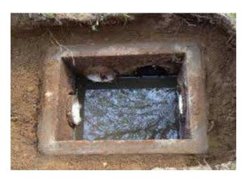
Three of the pipes from the distribution box are slotted pipes that sit on top of 750mm of sand (but under some crushed rock, topsoil and grass). These pipes are almost level so that they can distribute the effluent from the septic tank evenly over the sandy area.
