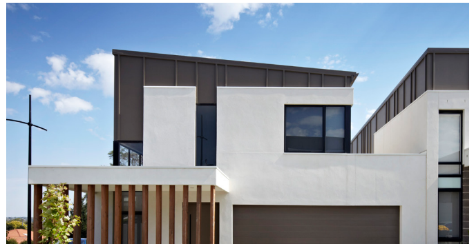
Skillion roof form combined with flat roof
