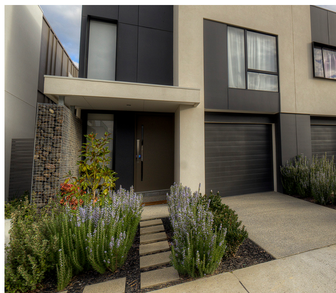
Recessed dwelling entry
