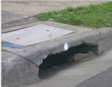
DE-005 Broken or missing pit covers
