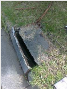
DE-005 Broken or missing pit covers
