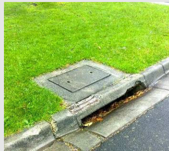
DE-006 Broken or missing pit grates including bike grates
