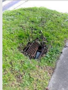
DE-008 Vertical displacement >25mm only if the pit is within a designated pedestrian walkway
