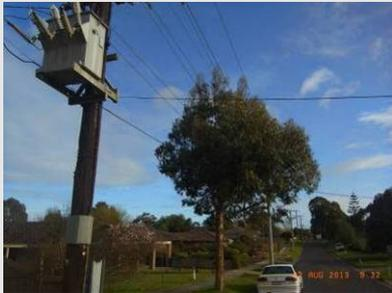
RV-002 Constructed Path Height Clearance < 2.5 m. Minimum 1m trafficable width on path with vegetation not exceeding 25mm in height representing a tripping hazard
