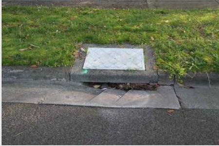
**DE-002 Pit throat (inlet) is damaged to the extent that it obstructs stormwater flow into the pit:**
