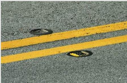
RS-008 Faded Statcon pavement marking (<50% effective reflectivity)
