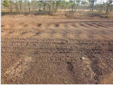
US-002 Potholes >500mm diameter and 150mm deep over 50% of the unsealed road or shoulder length
