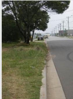
RV-005 Roadway Lateral Clearance < 200mm from back edge of shoulder and/or kerb
