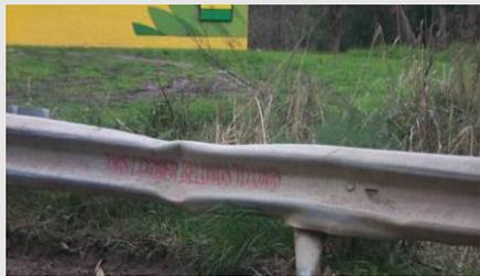
GR-002 Loss of >50% of guardrail reflectors
