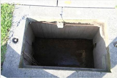
DI-004 Missing/ damaged/ deteriorated step irons and/or mesh panels.
