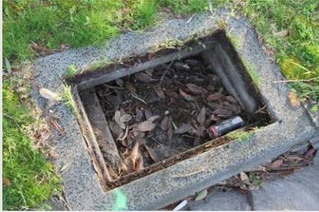
DI-002 Pipe/ culvert obstructions impede stormwater flow
