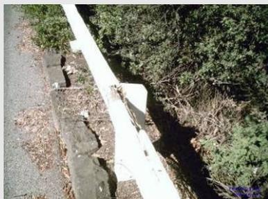
RF-002 Fencing posts, rails, strainers, wire or panels is not operational and is facilitating unrestricted access
