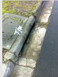
**DE-003 Lintel damaged or deteriorated to the extent that it could be hazardous to pedestrians**
