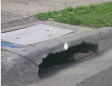
**DE-004 Reinforcement is exposed**
