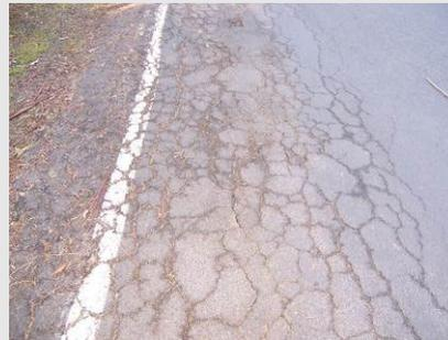
RS-005 Cracks >15 mm wide and covering an area of 5m<sup>2</sup> or greater
