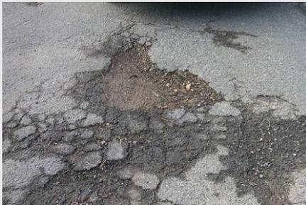
RS-004 Crocodile cracking with fines pumping
