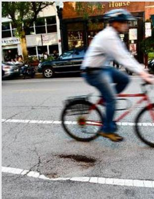
RS-002 Potholes >50mm deep and/or >150mm diameter in trafficable lane
