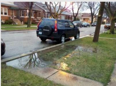
D-006 Water ponding over >60% of path for longer than 72 hours.
