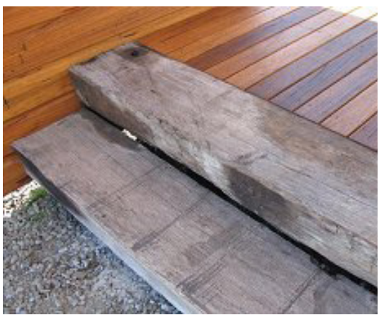
Ironbark decking with wharf timber edge
