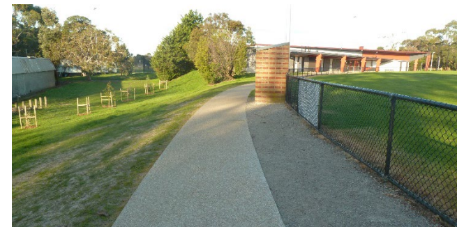
New exposed aggregate path to perimeter of Oval 1
