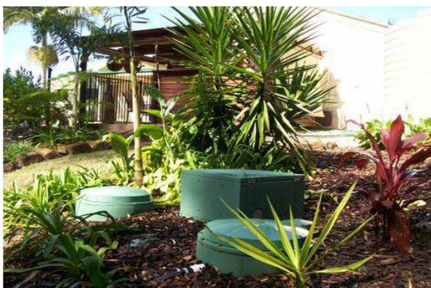
Treatment plants require a constant supply of electricity to operate, and a warning light or alarm that must be visible from habitable rooms in the house. The mechanical parts of a treatment plant (e.g. pumps, agitators, aerators, filters) require regular servicing every three months. This is an EPA
