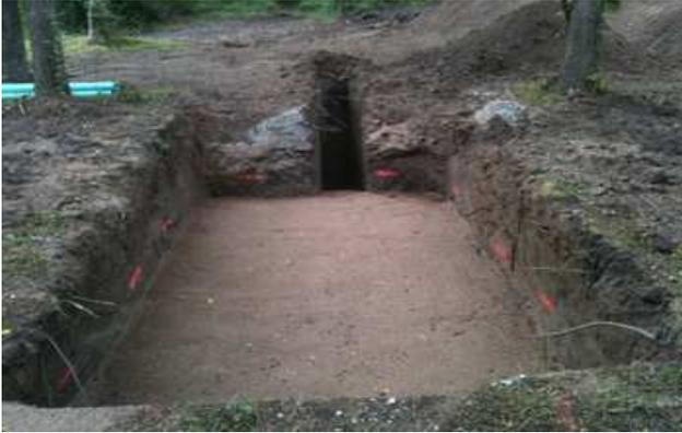
Three of the pipes from the distribution box are slotted pipes that sit on top of 750mm of sand (but under some crushed rock, topsoil and grass). These pipes are almost level so that they can distribute the effluent from the septic tank evenly over the sandy area.
