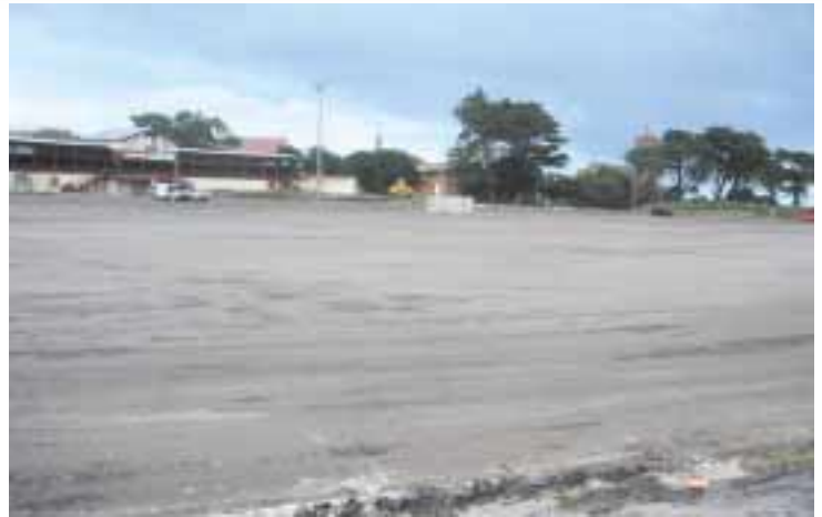
Ground renovations underway at Frankston Park
