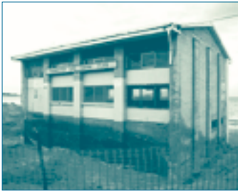
Life Saving Club under construction
